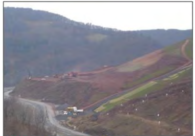
Prisms on the slope are used to monitor the slide.
