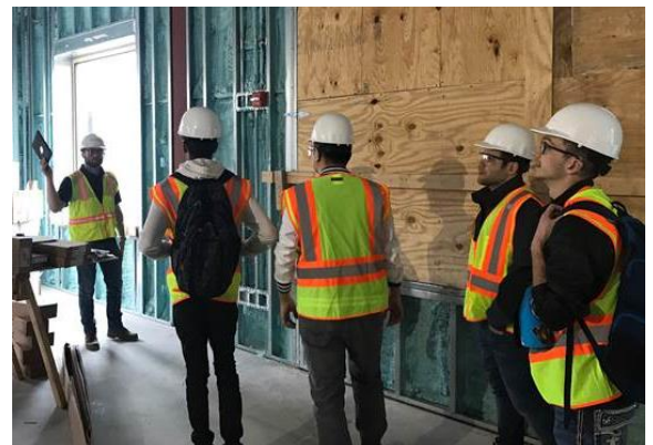
An interior tour of the New Steam Services Building
