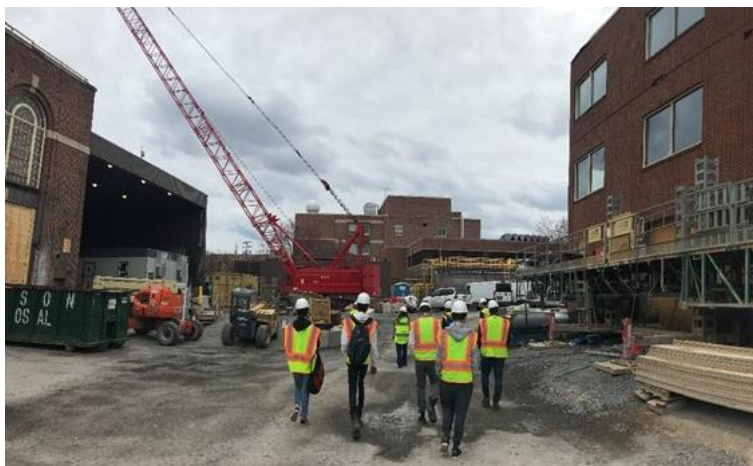
A walk around the perimeter of New Steam Services Building (right)
