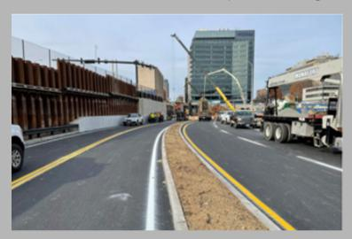
Downtown Crossing Phase 3 is a design-build project for the City of New Haven led by Manafort Brothers and PRIME AE Group. The design and construction included a grade separated connection of Temple Street over the new Service Drives to Congress Avenue, which will be connected via a future bridge, the Temple Street Bridge. The project was designed approximately 95% constructed within 12 months of notice to proceed including a 20-week scheduled closure of South Frontage Road.
