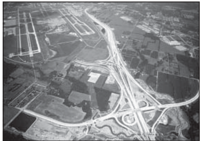
2005 Indiana Civil Engineering Project of the Year: I-70 "Fast Track" Interstate relocation project at the Indianapolis International Airport. Parsons Brinckerhoff Quade & Douglas was the lead design firm on the $170 million relocation and lowering of 4.5 miles of interstate highway.
