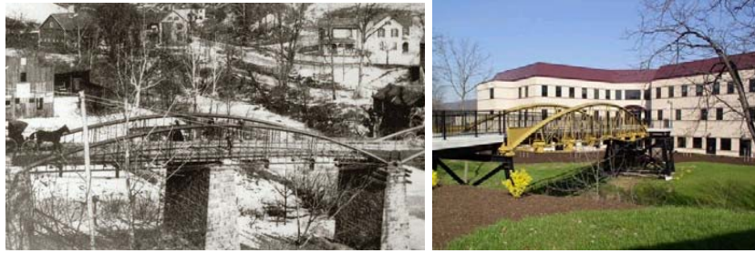
Pictures: Henszey's Bridge (1869), one of the first all-wrought-iron bowstring truss bridges, in its original home in Slatington, PA (left) and its new home at Central Pennsylvania College (right).
