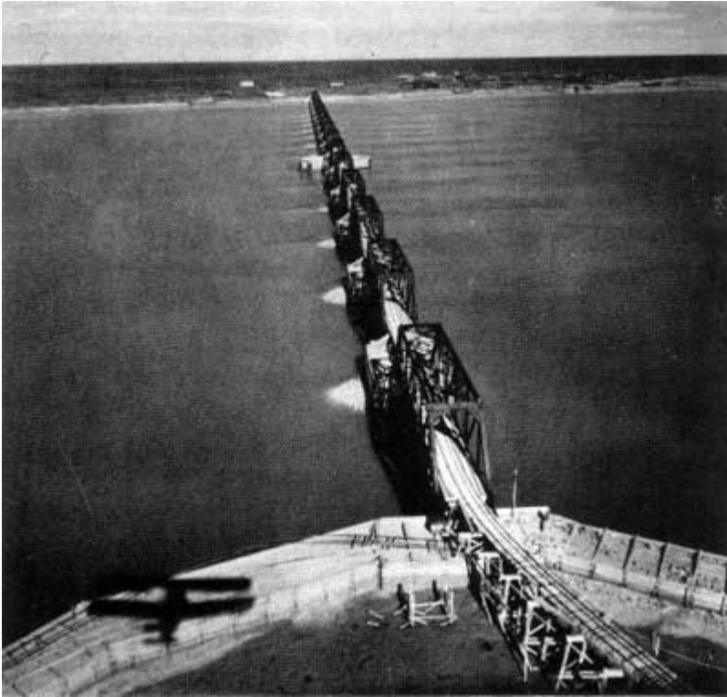
Figure 3. The half mile, 17 span bridge to the man-made island for the Port of Fort Nelson. Note the shadow of the biplane that took this photo, and the railroad tracks on the bridge.
