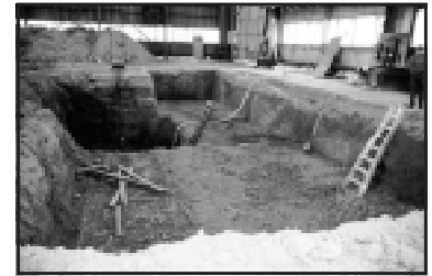
Figure 2: Excavation completed through stabilized ground, below groundwater level.
