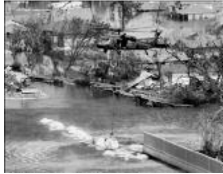
A Texas Army National Guard Black Hawk helicopter deposits a 6,000 pound-plus bag of sand and gravel into flood waters as work progresses to close the breach in the 17th Street Canal.
