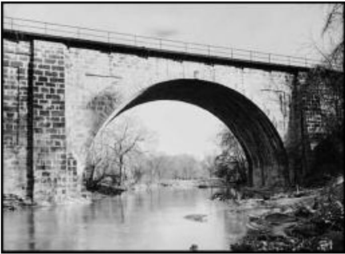
THE CARROLLTON VIADUCT Baltimore, Maryland Completed 1829
