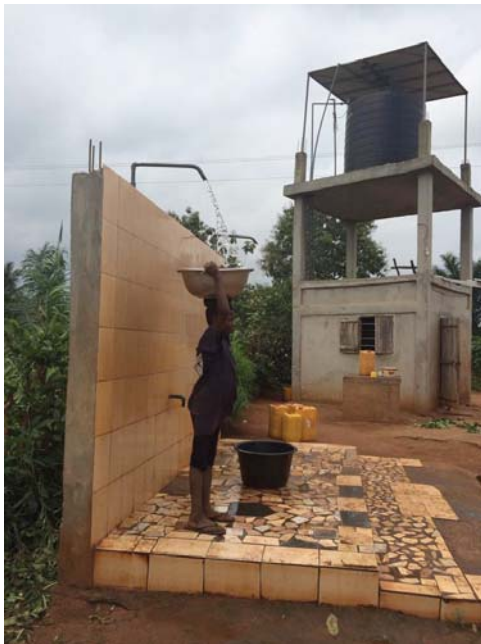
Figure 4. Photo of shallow water well (encased in concrete box in the background), elevated storage tank, and tap stand nearest to location of project.
