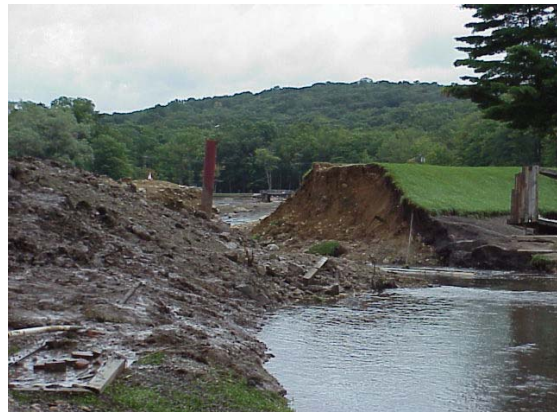
Tomahawk Lake Dam Failure – August 11, 2000 Sparta, New Jersey
