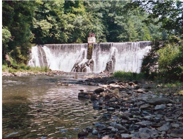
Lake Solitude Dam, Hunterdon County
