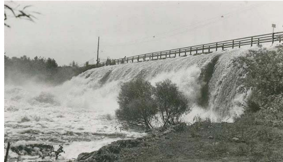
Union Lake Dam - Millville, New Jersey
