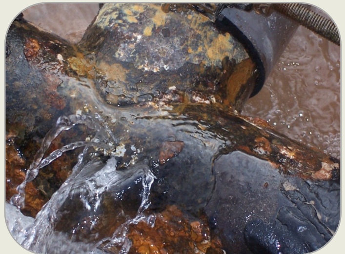
1950s steel line leak. Photo by J. Myers (11 May 2012)
