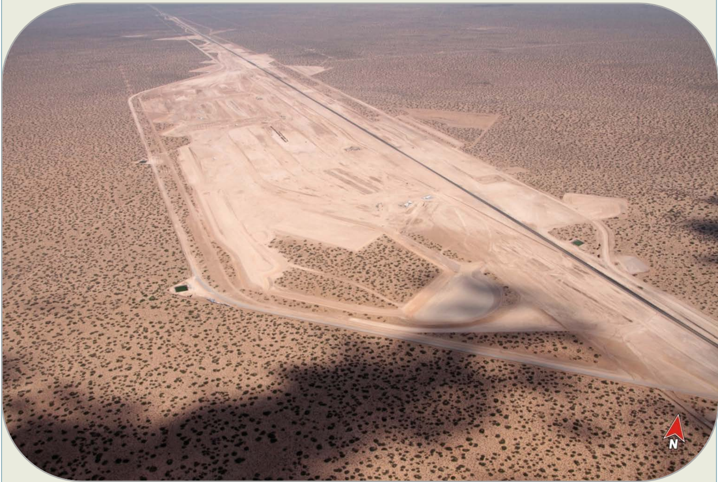
Photo of Strauss Yard, Union Pacific Railroad Sunset Route, under construction (May 2012).
