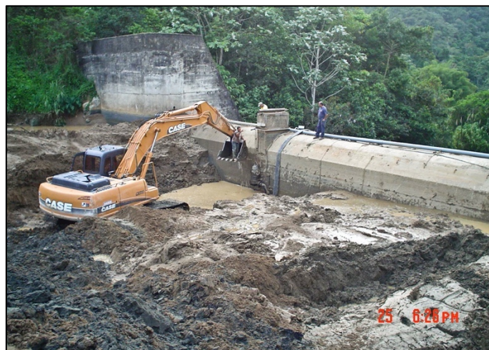
Figure 16: Sediment accumulation upstream of Pellejas dam.
