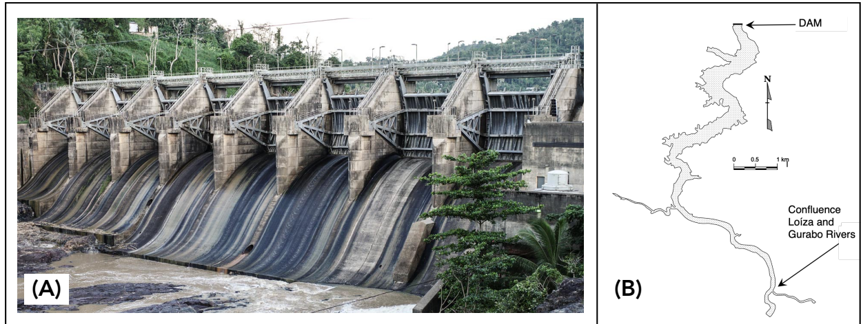
Figure 11: Carráizo reservoir showing: (A) large radial gates that extend to the full depth of the reservoir’s current storage, and (B) the elongated geometry favors the efficient transport sediment through the reservoir
