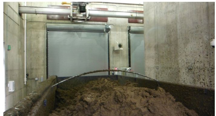
Solids Loading Area: One or two large truckloads of dewatered residuals, which are similar in feel to moist soil, are produced per week on average.
