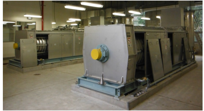
Screw Presses: Two screw presses each use a slowly rotating drum as the final stage of the solids dewatering system.
