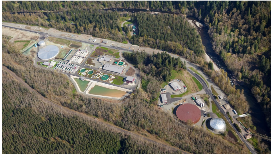
Aerial view of the Green River Filtration Facility.
