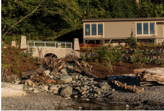
Restored North Creek connection to Seahurst Park shoreline. Opening the creek outlet to the beach restored the sediment delivery process from the bluff to the beach.
