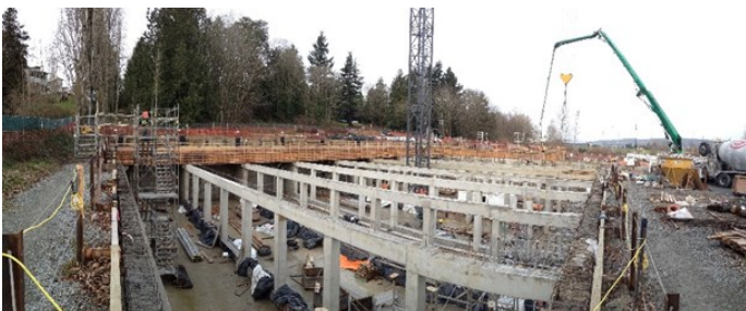
Windermere Combined Sewer Overflow Reduction
