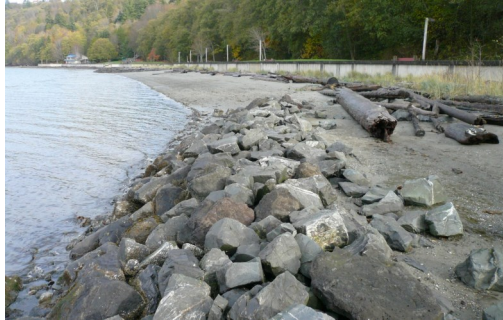
Left: Pre-project park shoreline with rock armoring and concrete bulkhead wall. The armoring and bulkhead were a safety hazard and degraded nearshore aquatic habitat.
