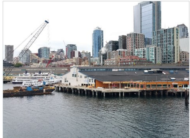
Photo 7: Pier 54 looking north. Note the retrofitted west and south aprons, the caisson lining area, and the revised window openings.
