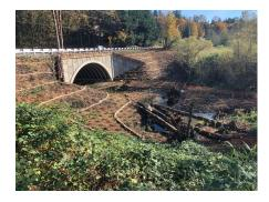
the composite arch bridge was used on the West Coast. It provided an elegant structural solution that was constructed more quickly and at a lower cost than other alternatives.
