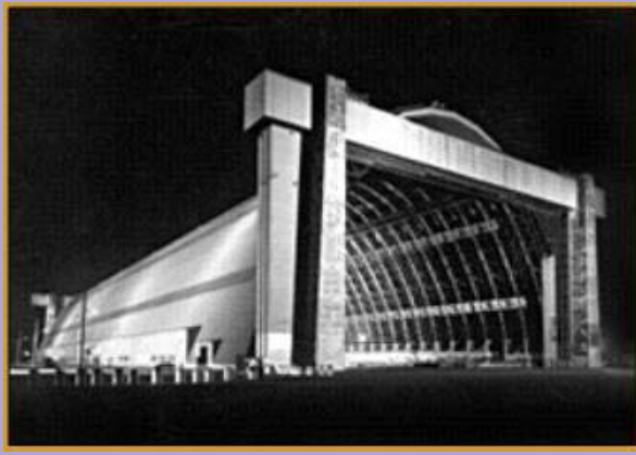
Blimp Hangar, Tustin, California Constructed 1942-1943
