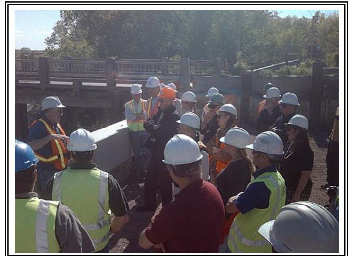
The group overlooking the Lime Kiln Bridge project.
