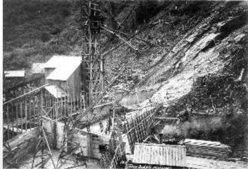
Figure 8 – Base formwork and early construction. Insley tower in place. (August 8, 1913)
