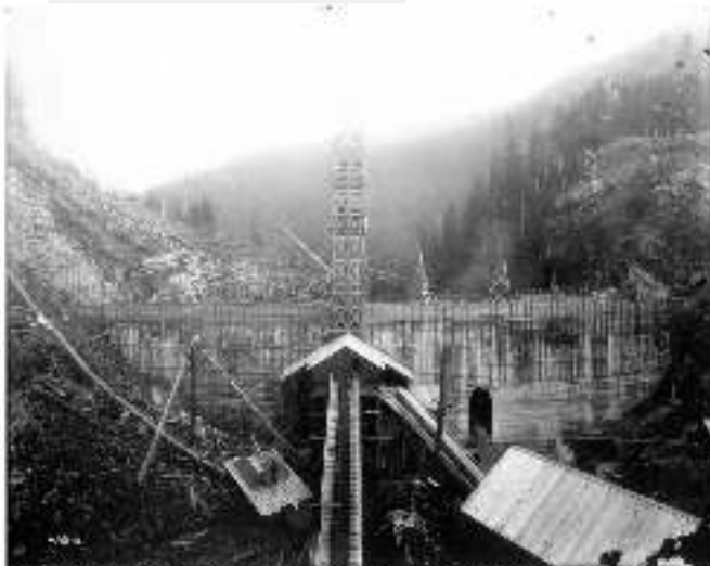
Figure 13 — Dam construction from upstream side. Tunnel conveyor to concrete mix house and Insley tower shown (September 25, 1913)
