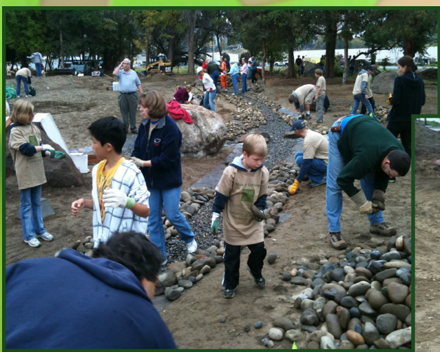
Volunteers Laying Rock Along the Creek
