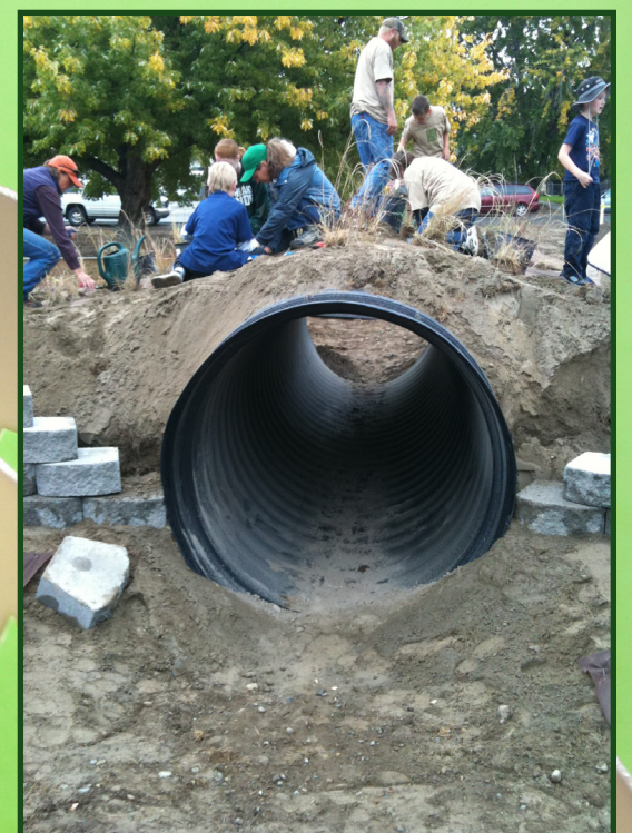
Prepping Tunnel for soft fall and Retaining Wall
