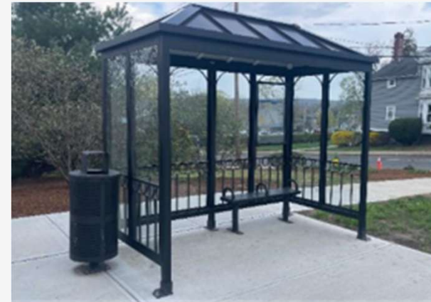
Waste Receptacle and shelter installed. Shelter roof style and grillwork customizations selected by the service area operator River Valley Transit to align with regional character
