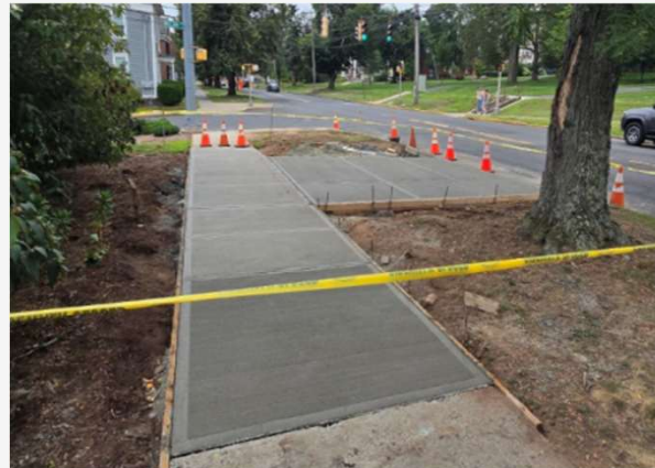
Finished concrete work, ready for shelter and amenity installation
