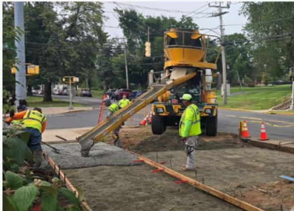
New concrete being poured for a shelter pad in Middletown, CT
