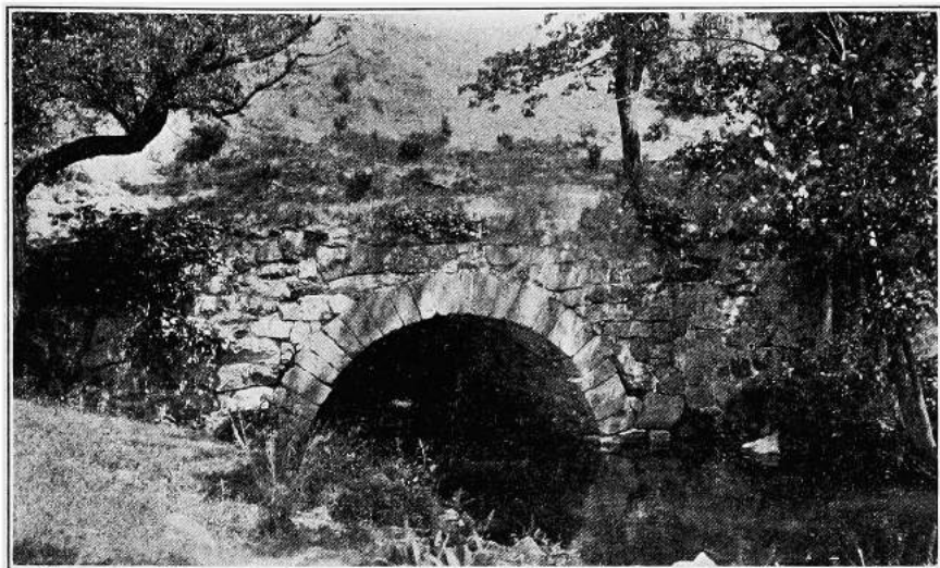
FIG. 5. TYPICAL STONE CULVERT UNDER CANAL.
