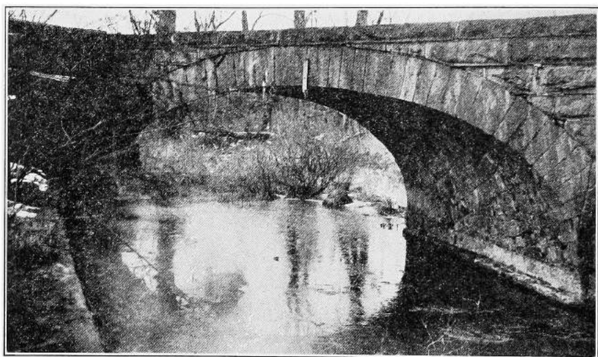
FIG. 7. SKEW ARCH CARRYING RAILROAD OVER CANAL NEAR BROOKSVALE, CONN.
