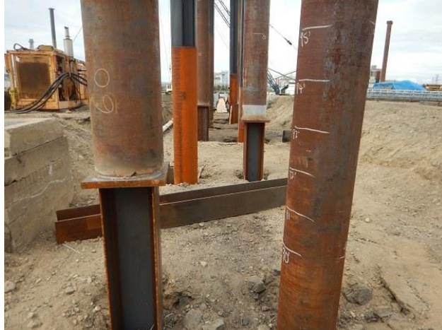
4 - H-Piles spliced with pipe piles for the deep foundation, extending approximately 130' into the ground.
