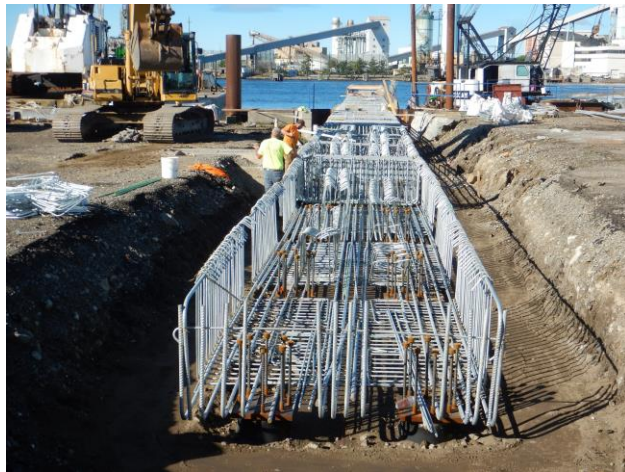
5 - Galvanized reinforcing used in pier foundation.
