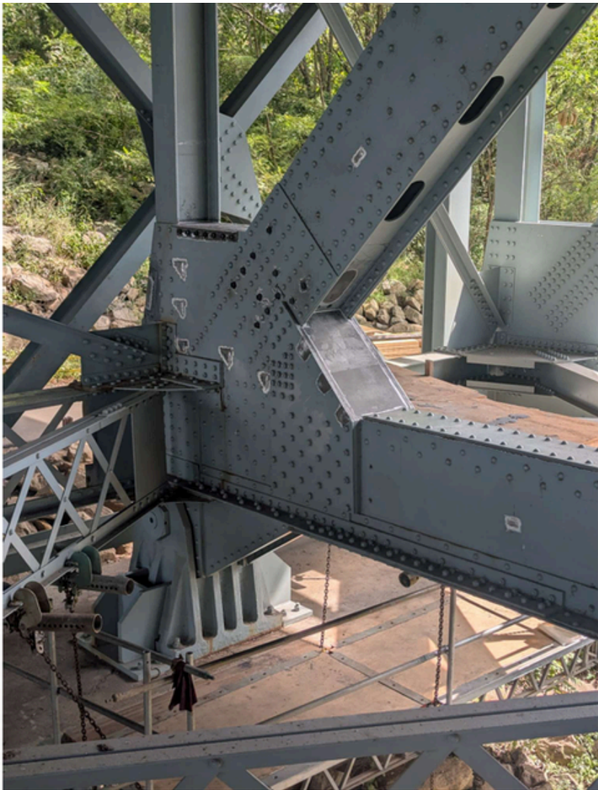
Completed UHPC Repair
