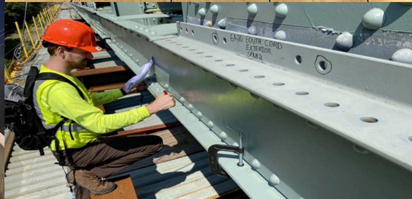
The numerous layers of paint on older steel bridges hide deterioration so during construction, inspection of the bridge continued.
