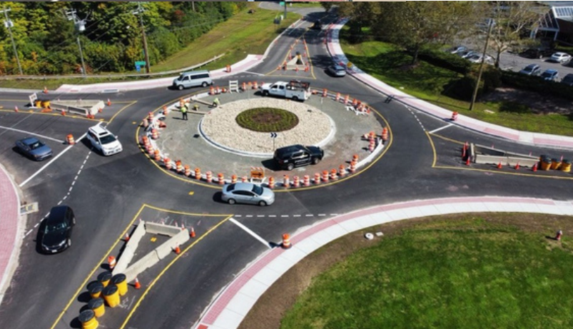
Construction of Truck Apron
