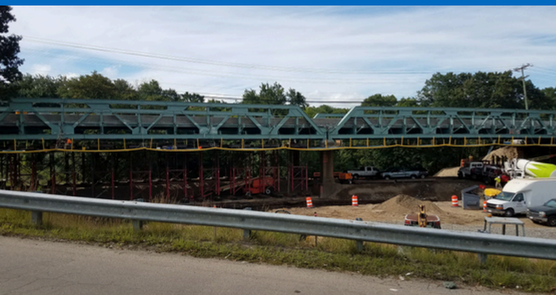
The design of Bridge No. 00488 incorporated full support for the truss bridge throughout construction, providing uninterrupted service.
