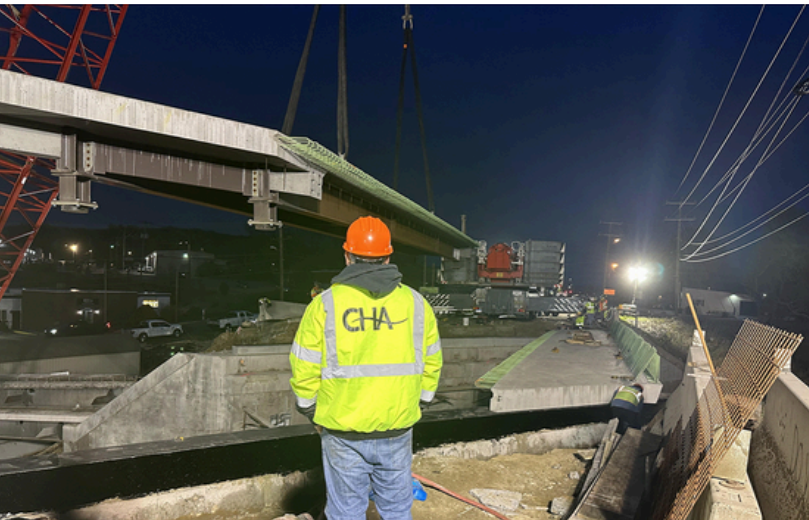
The superstructure replacement of Bridge 00489 utilized prefabricated bridge units put in place over a single weekend.
