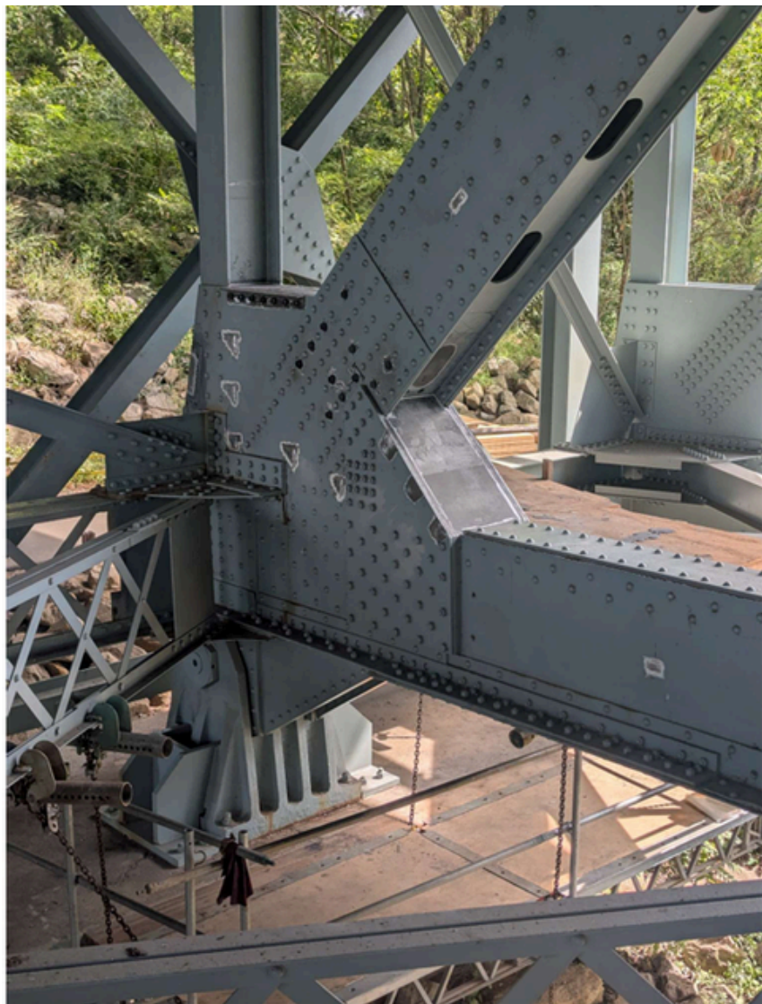
Completed UHPC Repair
