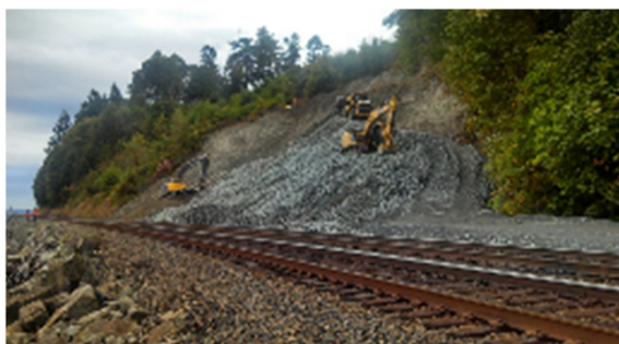
Railroad landslide mitigation, Snohomish County
