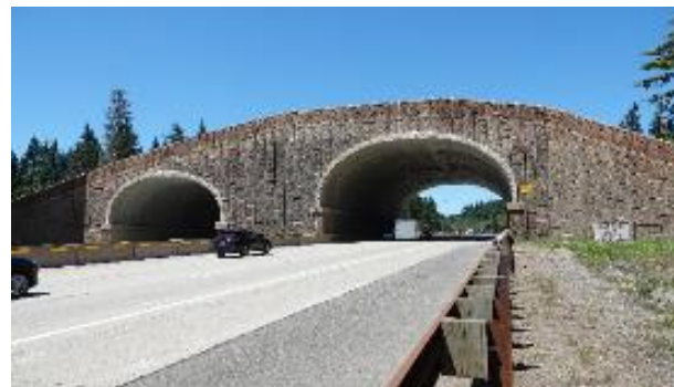
I-90 improvements/ wildlife crossing
