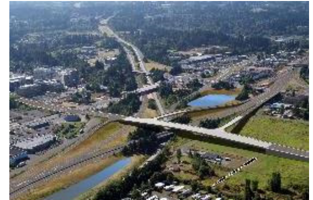
Salmon Creek I-5/I-205 interchange
