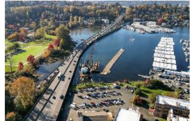
Portage Bay Bridge and Roanoke Lid project
