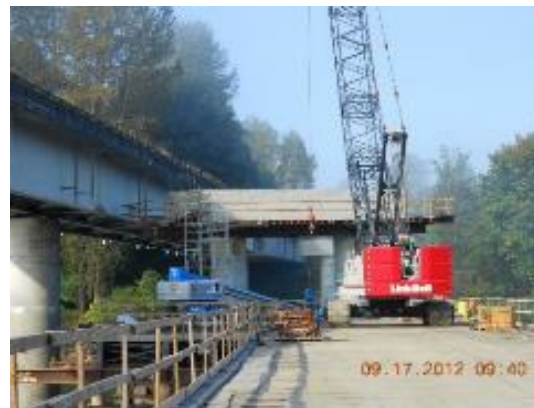
SR 522/Snohomish River Bridge widening
