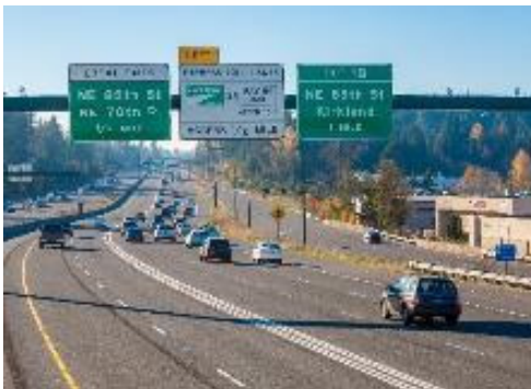
I-405 Express Toll Lanes
