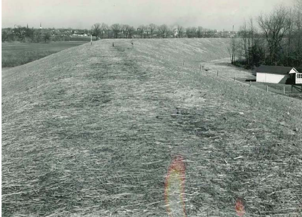
Figure A.3 – The Louisville Levee As Construction Was Completed in 1948 This project has 67,321 lf of earth levee.
