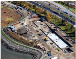
intercepting flow from existing CSO outfalls and sending it to a new 3.5 million-gallon (MG) offline CSO storage facility. The City's goal is to reduce the annual overflow volume from CSO outfalls 16, 17, and 18 from 150 MG to approximately 18 MG. The project is being constructed as a design-build project. As the design-build lead, Sargent Corporation is managing
