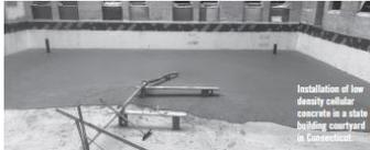
Installation of low density cellular concrete in a state building courtyard in Connecticut
