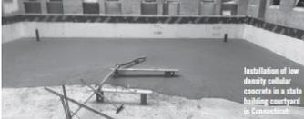
Installation of low density cellular concrete in a state building courtyard in Connecticut
