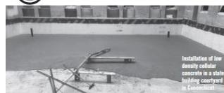
Installation of low density cellular concrete in a state building courtyard in Connecticut
