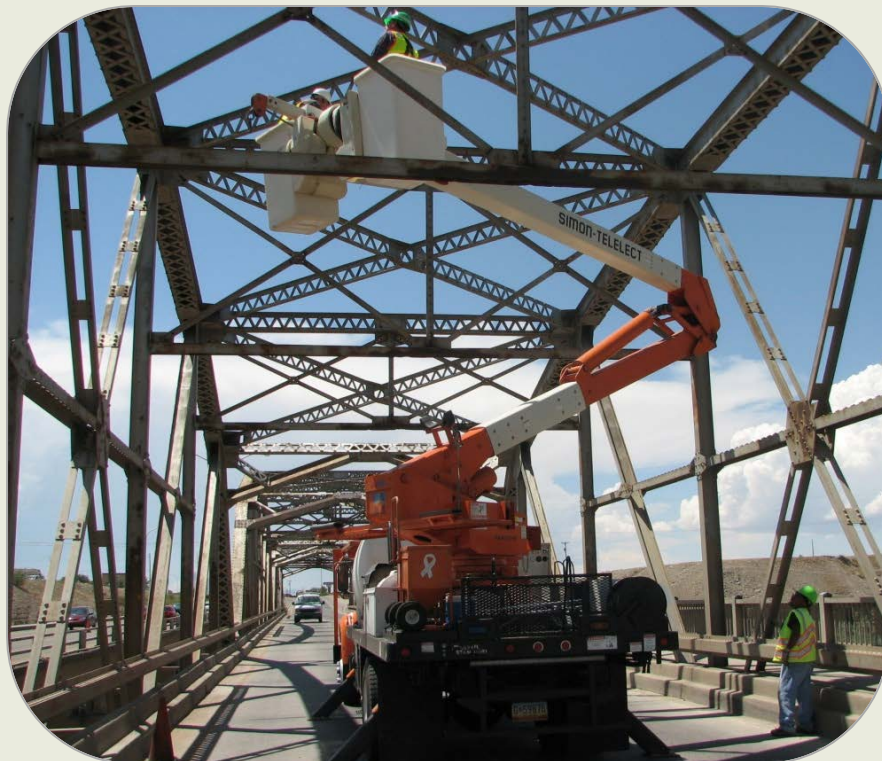
Safety inspection of complex truss bridge.
