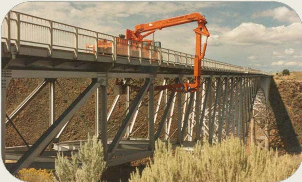
Inspection of the Rio Grande Gorge Bridge.
