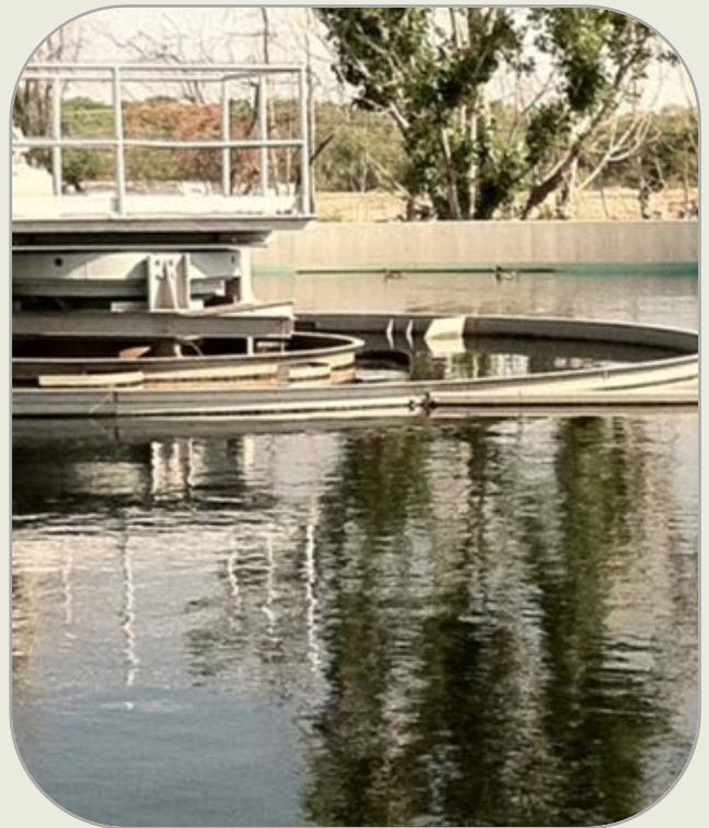
Primary clarifier (solids at SWRP settling). WUA photo (no date).
