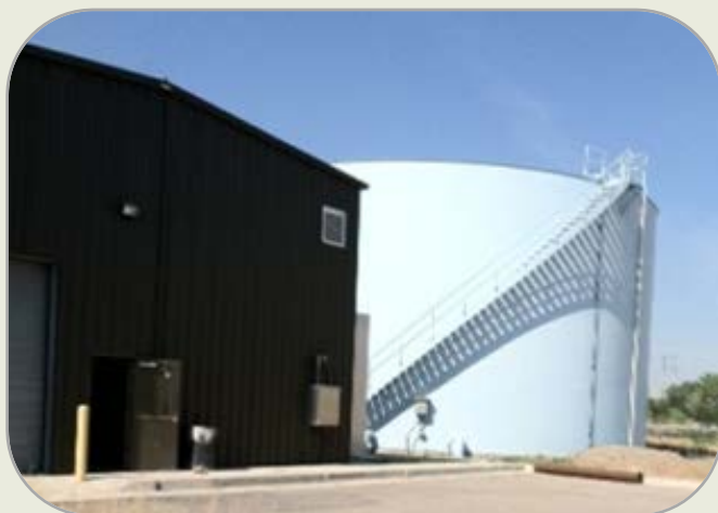
Old reuse tank at SWRP. WUA photo (no date).
