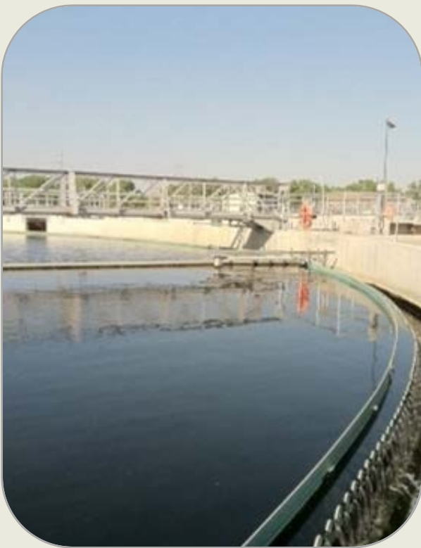
Final clarifier at SWRP. WUA photo (no date).
