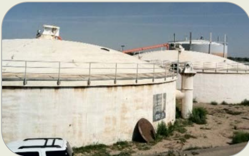
Anaerobic digesters at the SWRP. WUA photo (no date).
