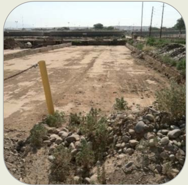
Sludge drying bed at SWRP. WUA photo (no date).
