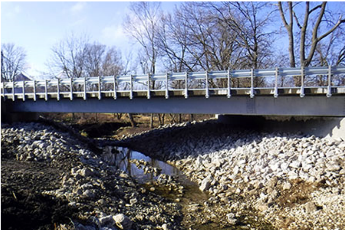
Photograph Number 1: New bridge carrying Evans Mill Road over Hickory Run Creek
