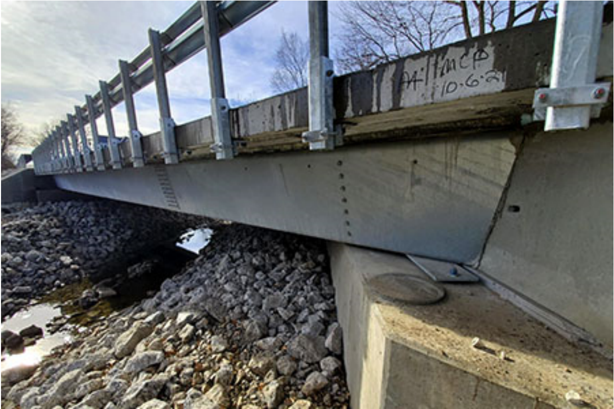
Photograph Number 2: Installed Pre-cast Deck
