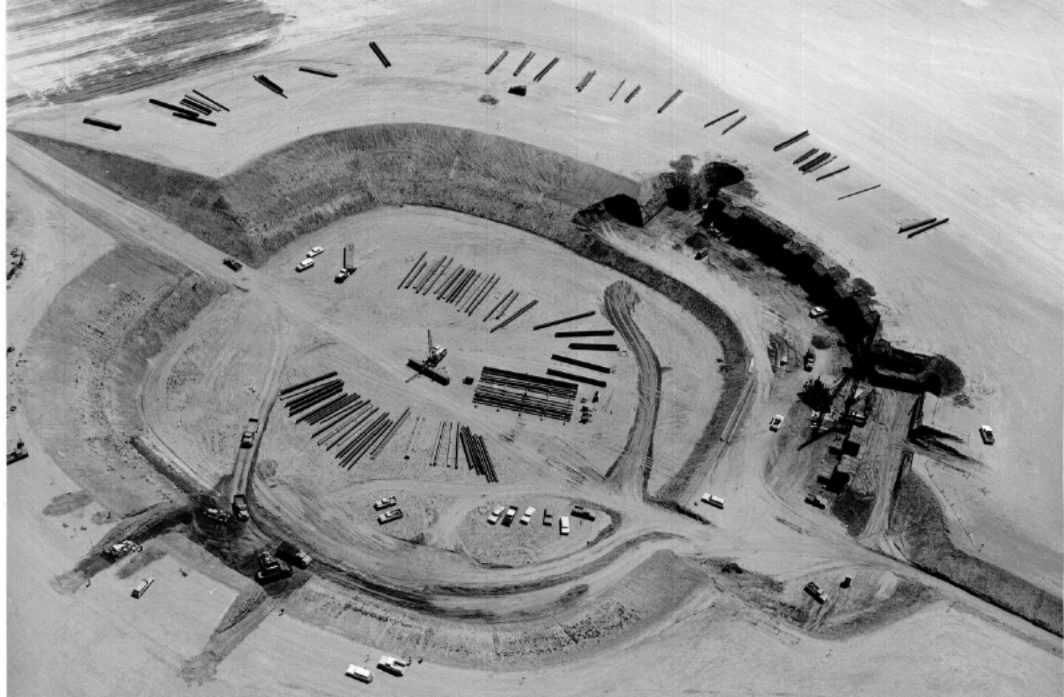
APRIL 26, 1966 - CITY-PURCHASED PILING DELIVERY ON SITE COMMENCED APRIL 8, 1966. THE PILING CAN BE SEEN STOCKPILED RADIIALLY ABOUT THE STADIUM AND ON THE STADIUM FLOOR.
