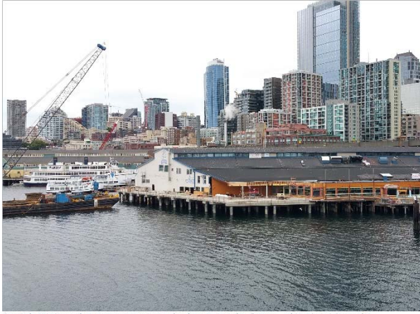
Photo 2: Pier 54 looking north. Note the new, recycled steel and south apron, the outdoor dining area, and the revised window openings.
