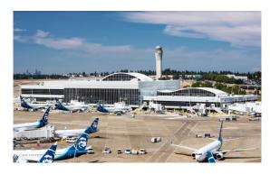
seismic upgrade and all new building mechanical systems. The project added eight new aircraft gates (for a total of 20), new PCC commercial apron areas, Alaska's flagship lounge, hold rooms, a renovated transit station, concessions, art, expanded baggage handling, and airline/airport offices and support spaces.
