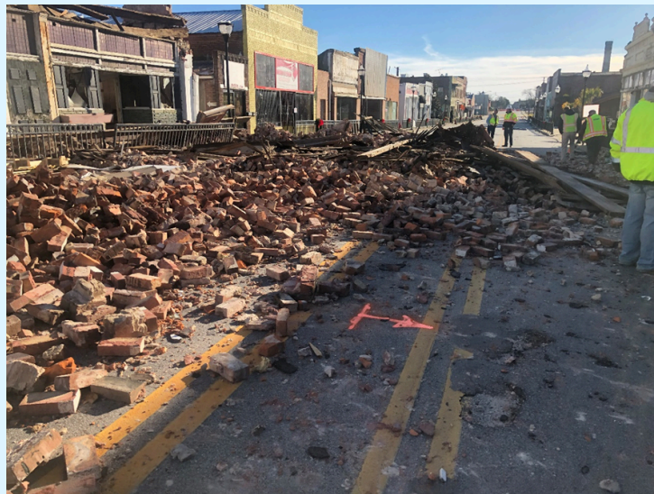
Downtown Bamberg Tornado Recovery (JLA)
