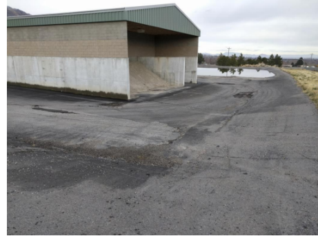
Figure 1: Storage structure, collection swale, and retention pond,
