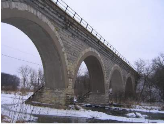
Modern Day Bridge Photo Showing Shotcrete Arch Reinforcement from 1930
